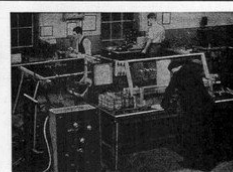
METER TESTING DEPARTMENT
